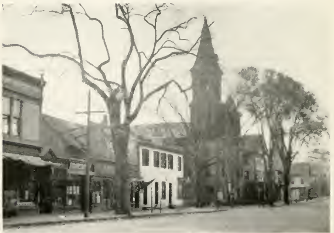
STREET VIEW SHOWING THE BAPTIST CHURCH IN WHITMAN, FORMERLY SOUTH ABINGTON MASSACHUSETTS
